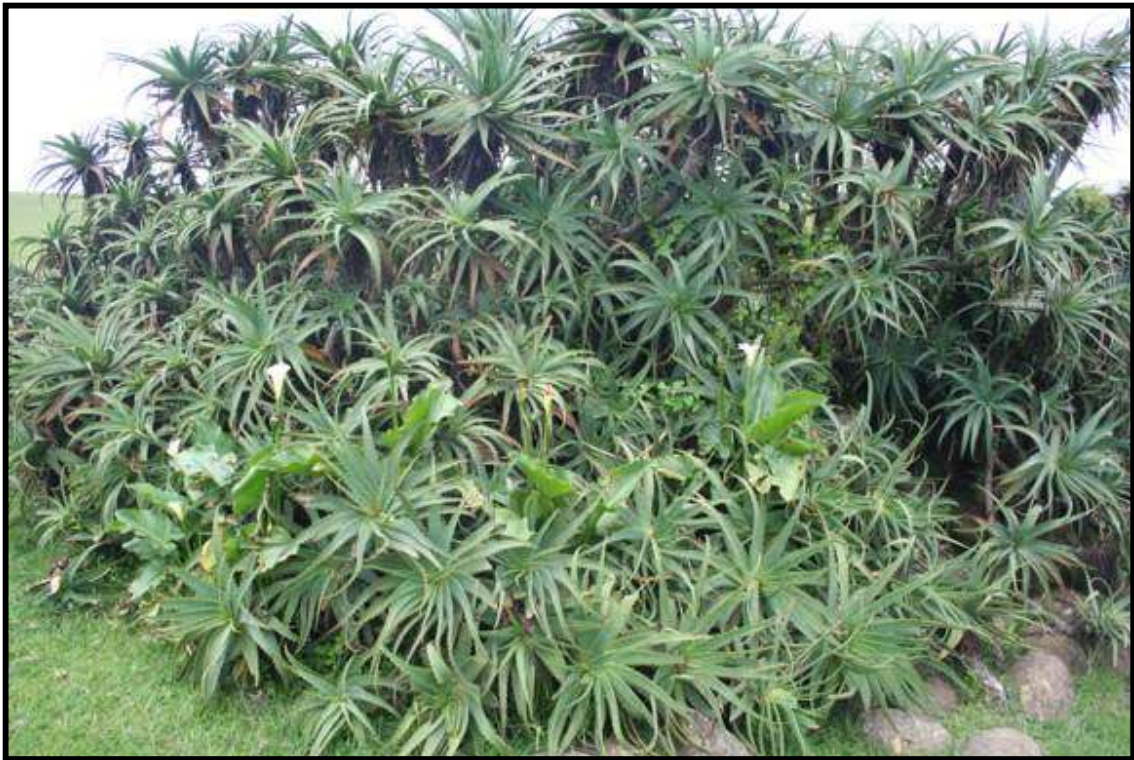
FIG. 36: DENSE VEGETATION ON THE STONE WALLING AT N66
