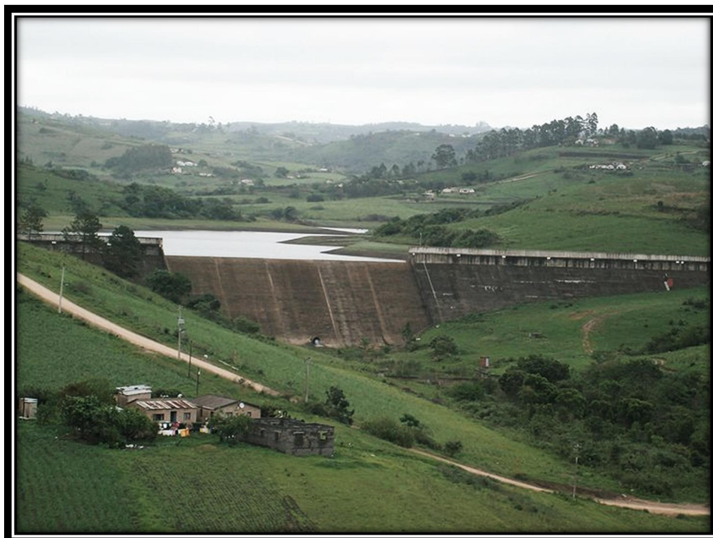
Figure 2. The proposed Nungwane Raw Water Pipeline start at the Nungwane Dam and runs east towards Amanzimtoti.
