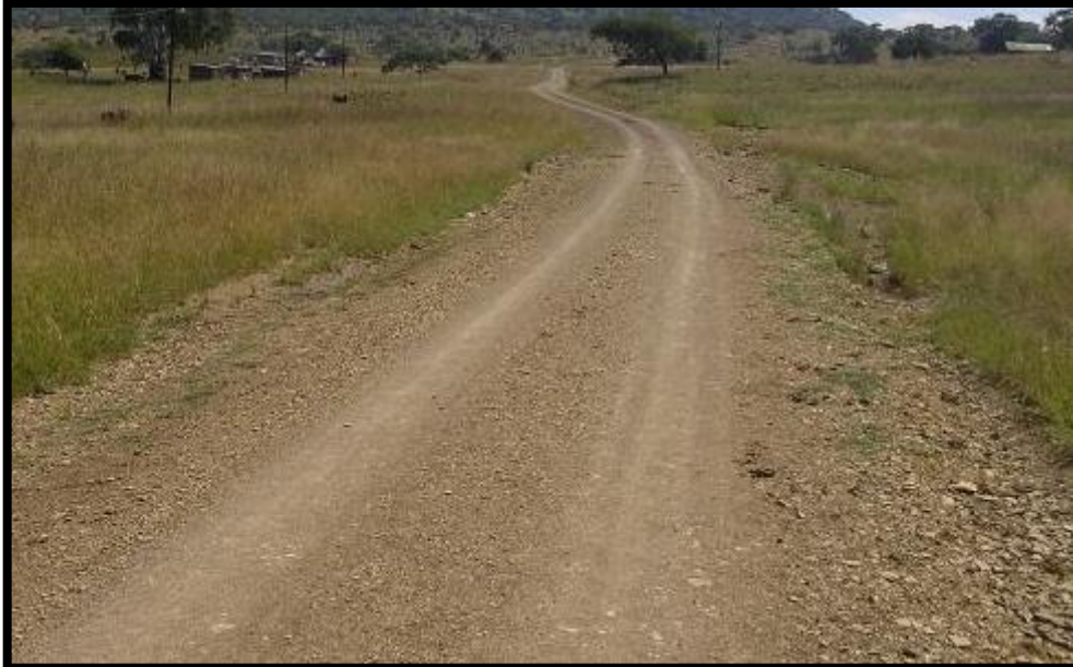
Figure 2. The D 1291, a gravel road that connects with the proposed access road.
