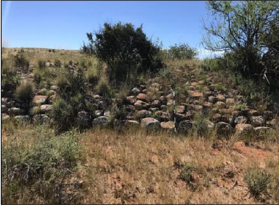
Figure 31: Stone clad dam wall at PL_05 (Mann 2022: figure 73).
