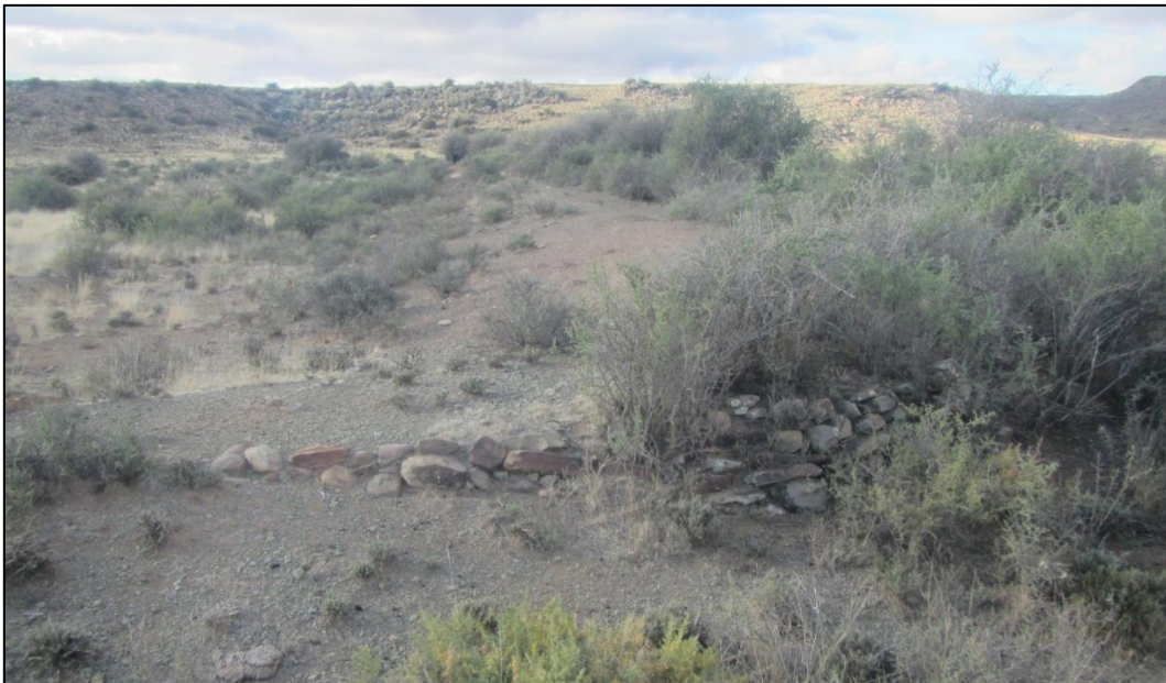
Figure 32: Low earthen dam wall (running away from the viewer) with a section of stone walling lining the spillway at waypoint 203.
