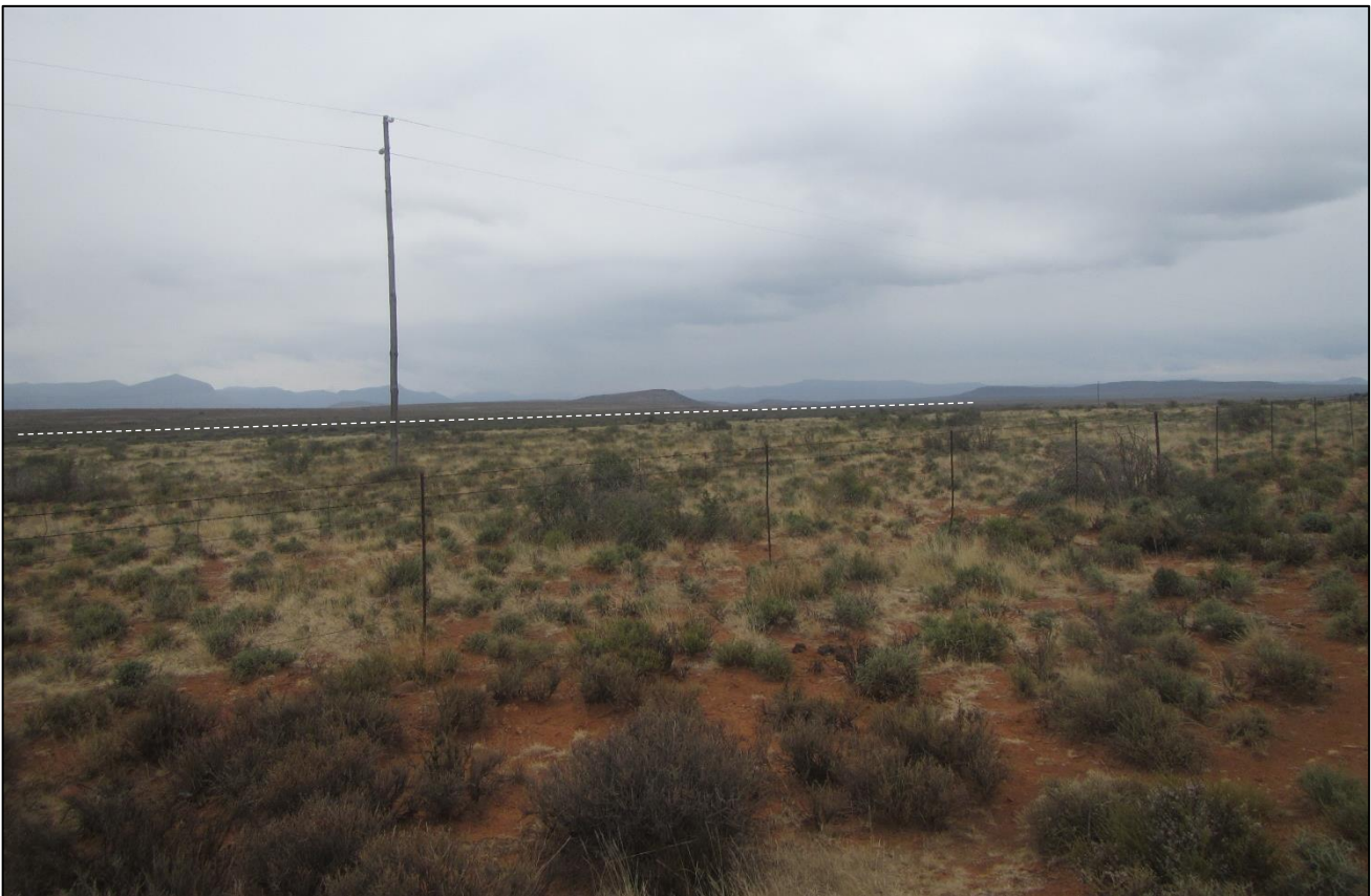
Figure 12: View towards the south towards the southeastern end of the powerline. The white dotted line indicates the approximate alignment of the proposed powerline.
