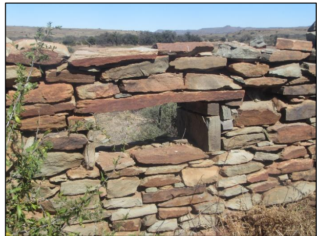
Figure 21: Window at waypnt 214.
