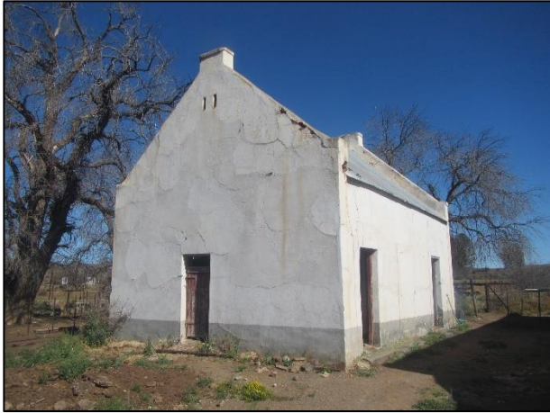
Figure 29: The small historical structure at waypoint 205.
