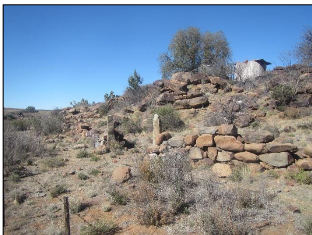
Figure 16: Stone walling built around a rocky hill to create a kraal.
