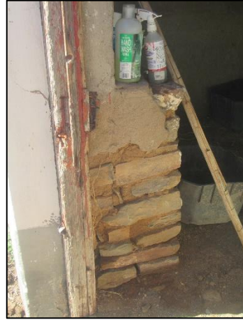
Figure 30: Thick stone and mud mortar wall inside the structure at waypoint 205.
