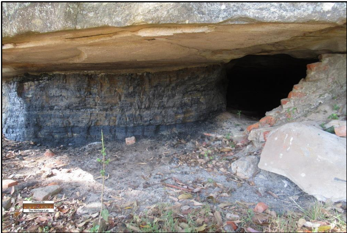
Figure 6. One of the adits of the old coal mine. (These adits were closed off with bricks, but all of them have been broken open again, probably by people looking to extract some coal – see the poor quality seam at the bottom of the entrance)
