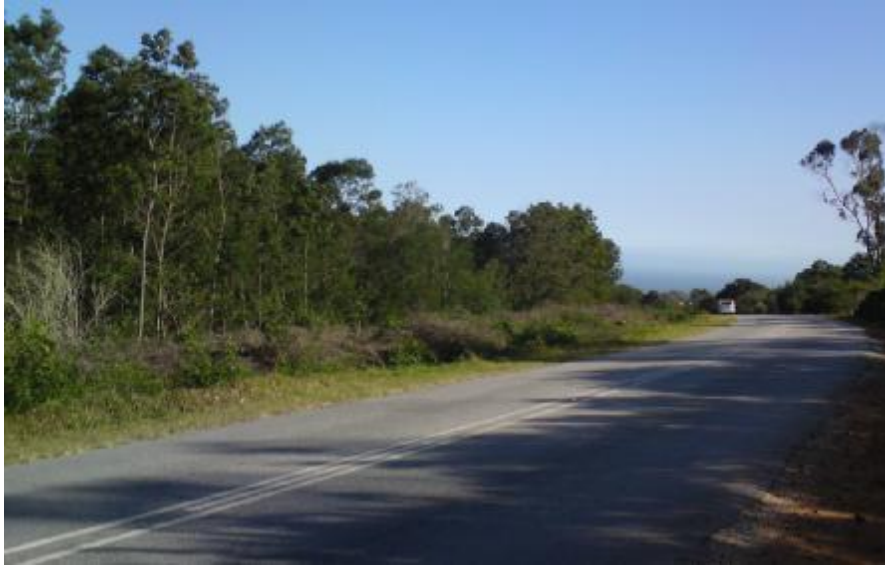
Figure 3: The site on the left seen from Seaview Road (M9)
