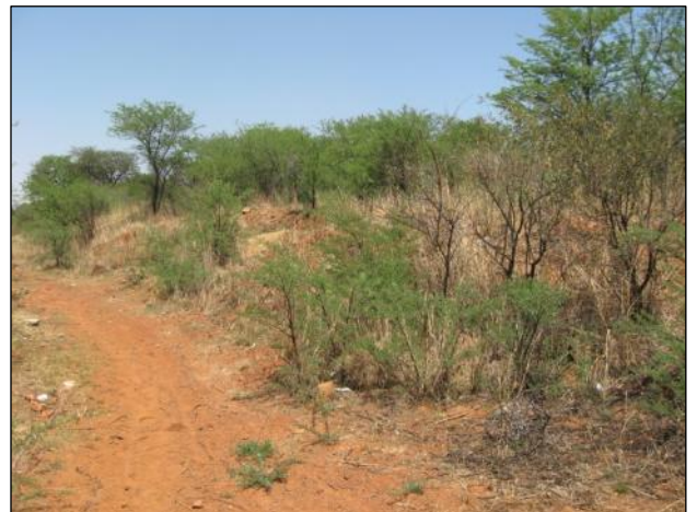
Figure 7 – View of berm along the eastern boundary.
