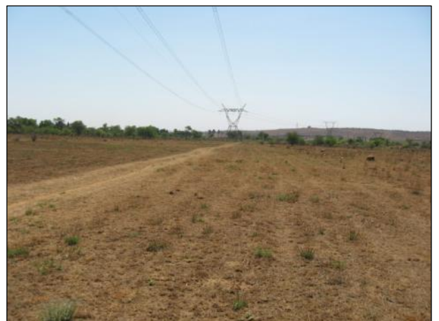
Figure 9 – One of the power lines across the site.
