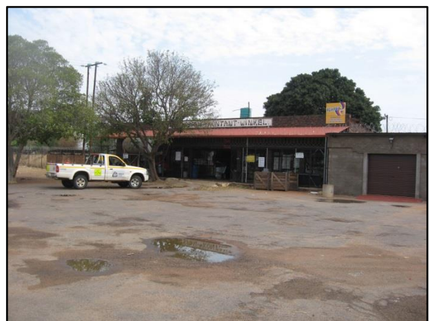
Figure 9 – View of the shops adjacent to the D175 Steenbokpan – Stockpoort road.
