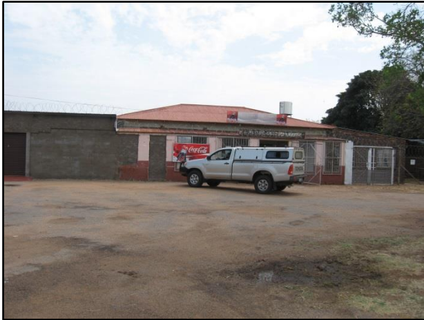
Figure 16 - View of the identified shop with some of the later modifications.
