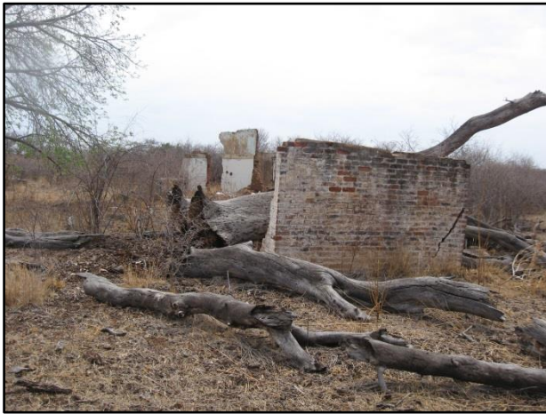
Figure 13 - General view of the dilapidated structure from the west.
