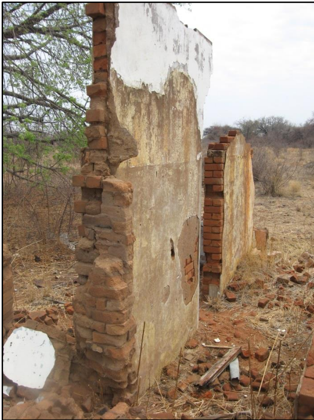
Figure 15 - View of the clay and mud bricks in the walls.
