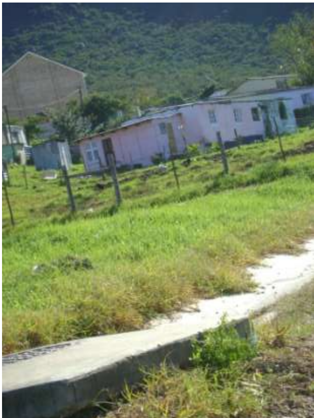
Existing Infrastructure – Storm water drains
