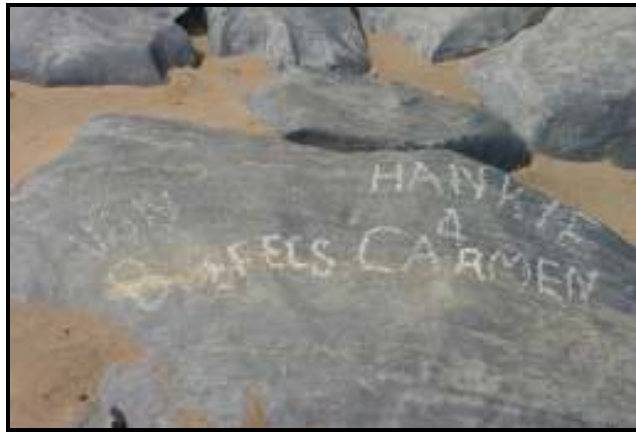
Figure 79: Graffiti impacting on Site BLD28
