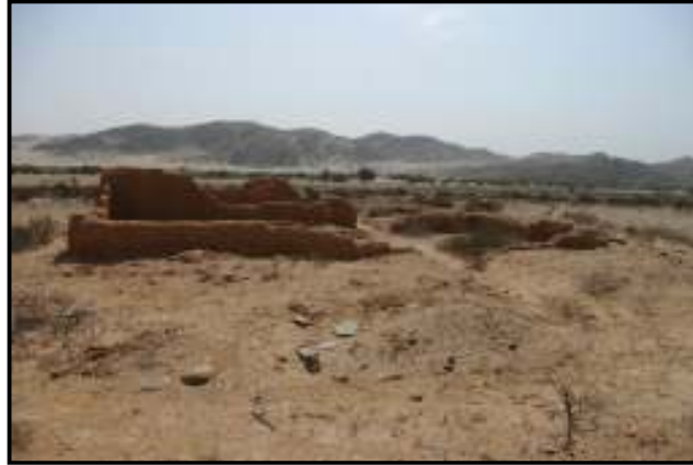
Figure 25: General view of Site B3
