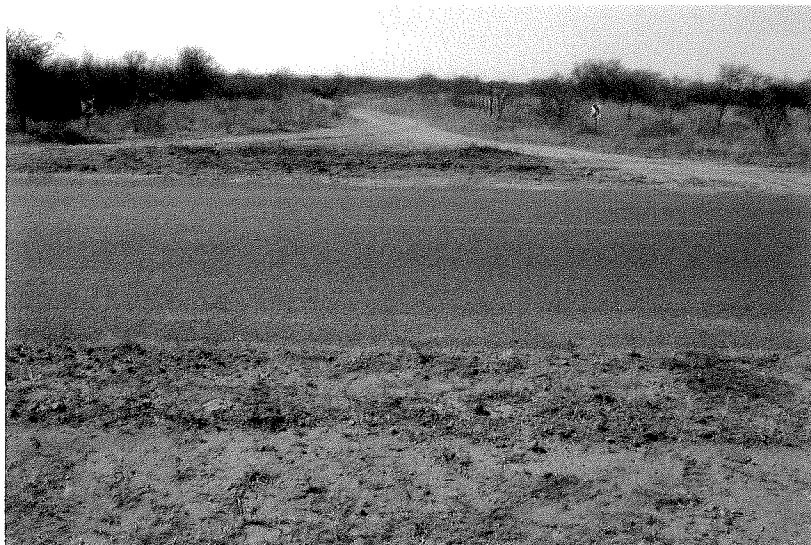
Figure 1: View of the starting point of road D2740
