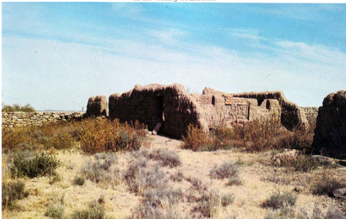
Figure 8. The “kleihuis” ruins at Klipplaatsdrif built ca the 1830’s, one of the earliest Trekboer dwellings north of the Orange River.
