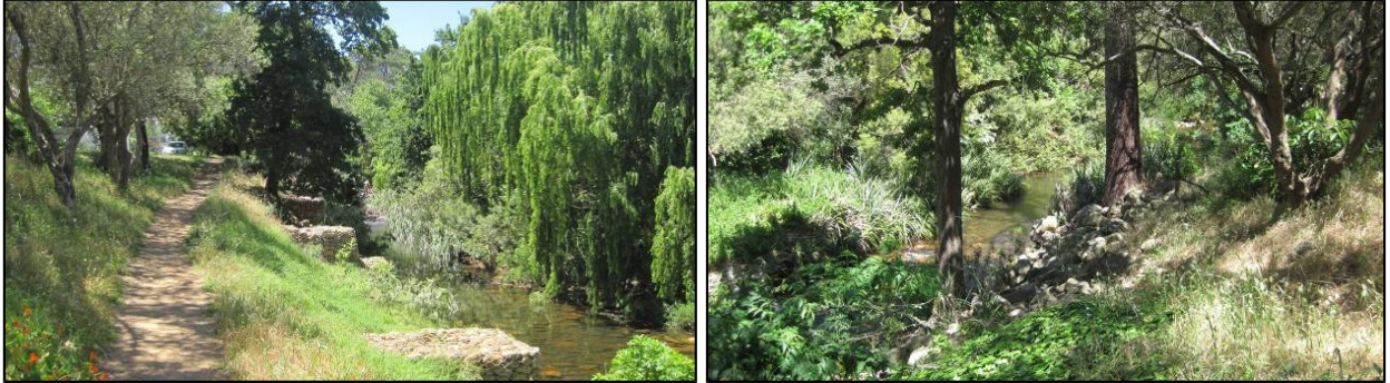
Intervention site 300-001 gabions (existing can be seen at left), Intervention site 300-002 tree roots
