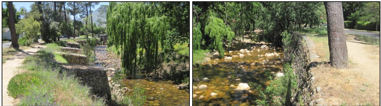
Intervention site 300-003 (l&r) existing gabions and retaining wall
