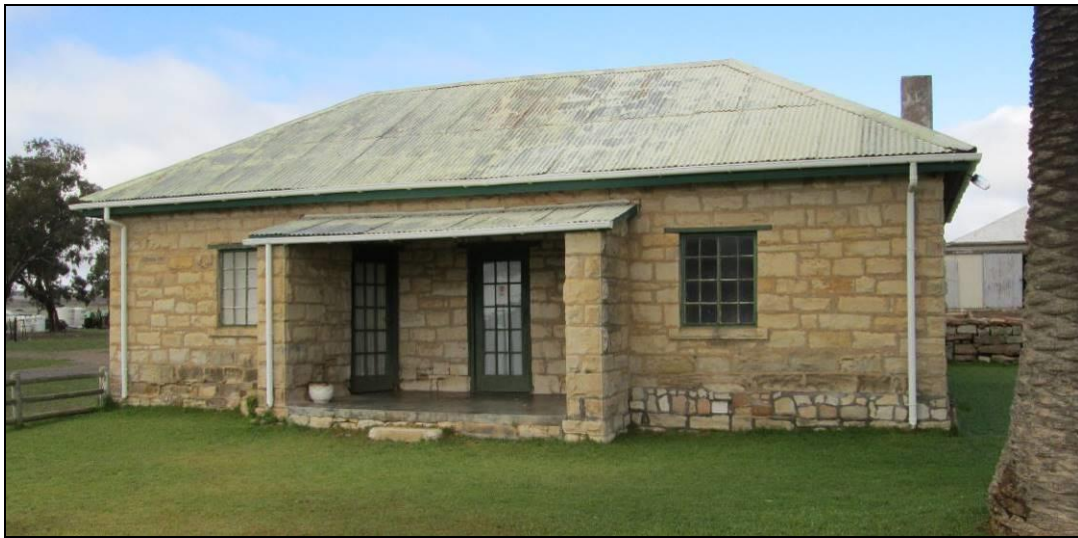
Figure 16: View of the north elevation of the stone house.
