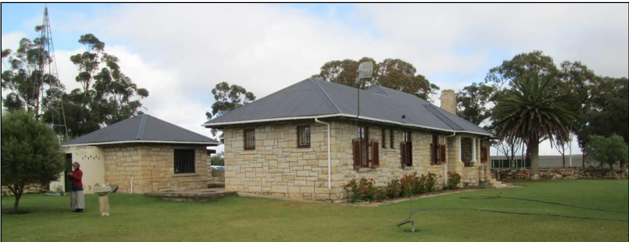
Figure 15: View of the north-eastern corner of the administration building. The small store room is visible to the left.
