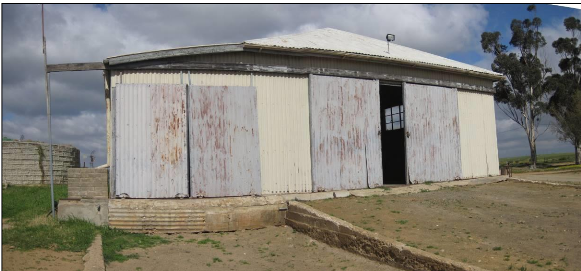
Figure 20: View towards the south of the corrugated iron shed that predates 1951.
