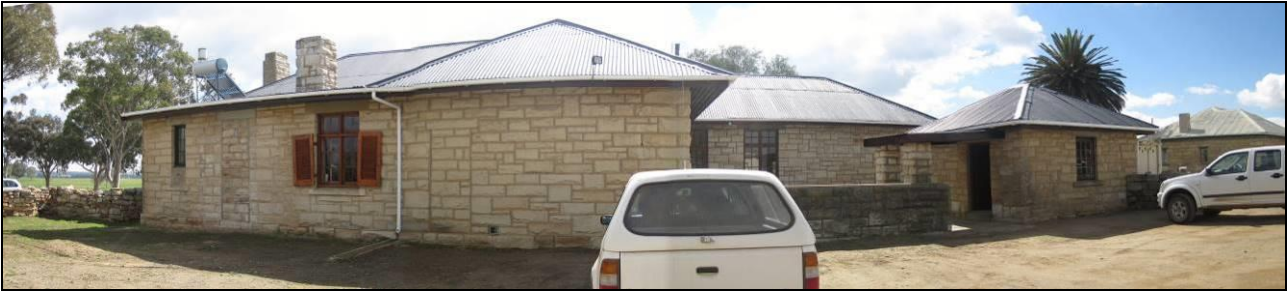
Figure 14: View of the southern elevation of the main admin building. Two closed up doorways are evident to the left in this view. The small store room is visible to the right. Photograph: Kirsty Robinson (SEC).
