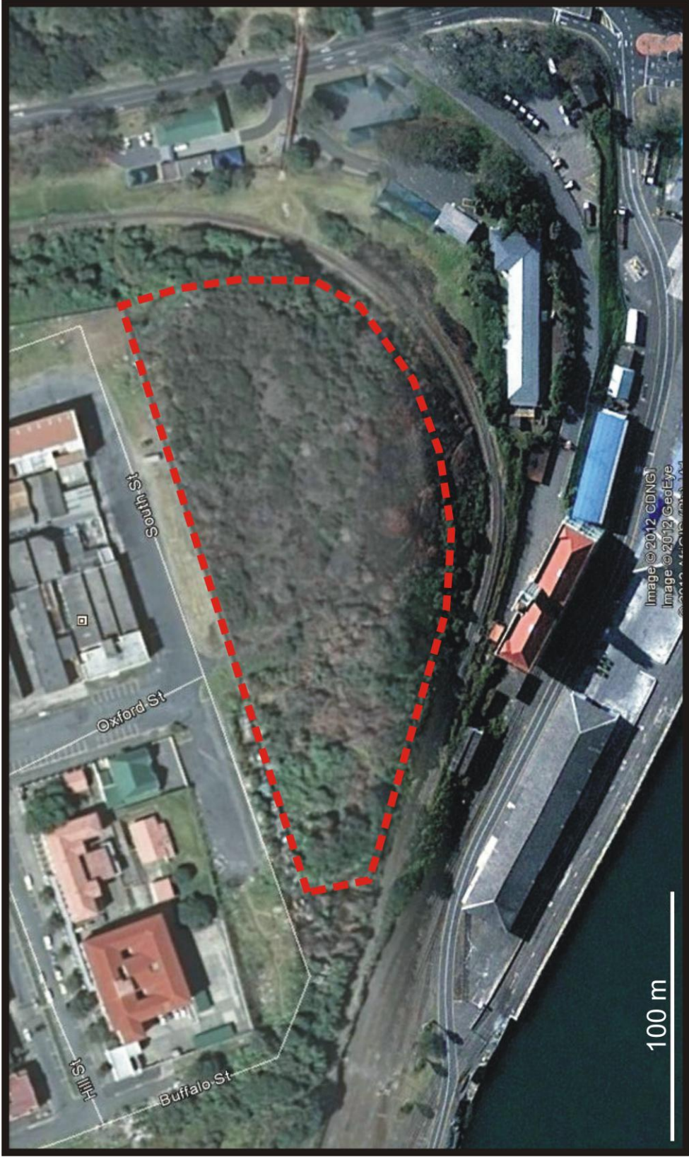
Figure 2. Aerial view of the proposed site.
