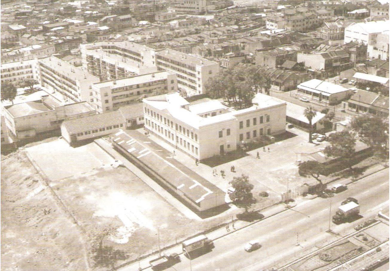
Figure 17: Aerial view: Harold Cressy High School circa 1994 before alterations and additions Note prefabs located along Roeland Street, along McKenzie Street and across the current quad (Victor John Ritchie collection)
