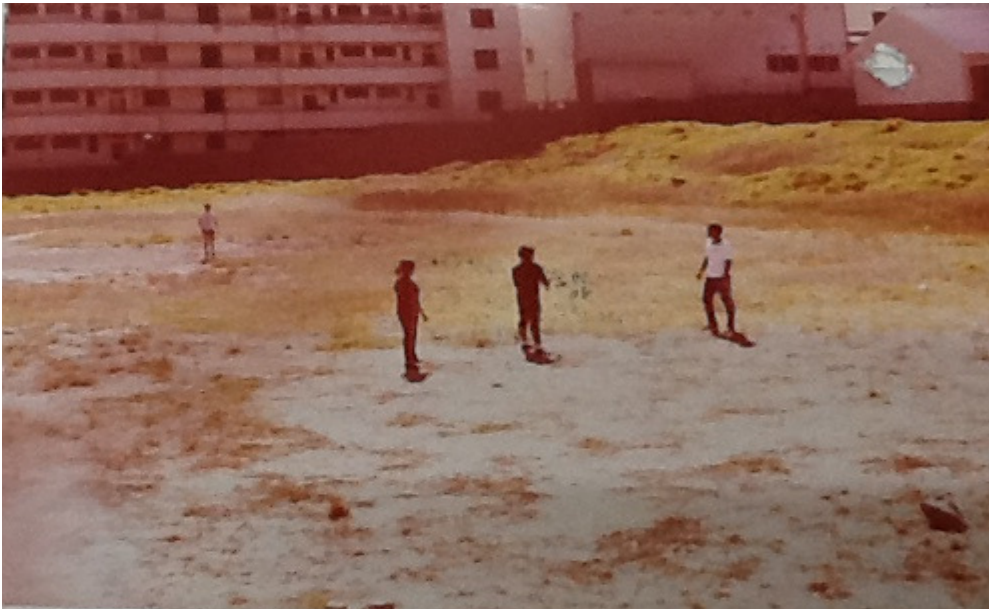
Figure 15: Surface of the playgrounds in poor condition circa 1983 (National Archives)
