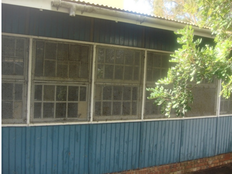
Figure 11: Prefabricated classrooms on the border of Roeland Street
