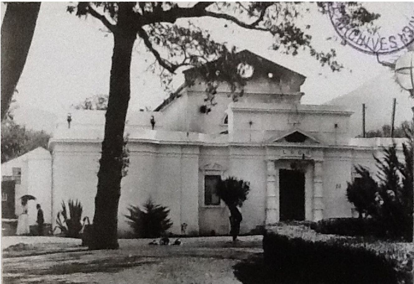
Figure 10: Good Hope Lodge after the fire (National Archives E 6320)
