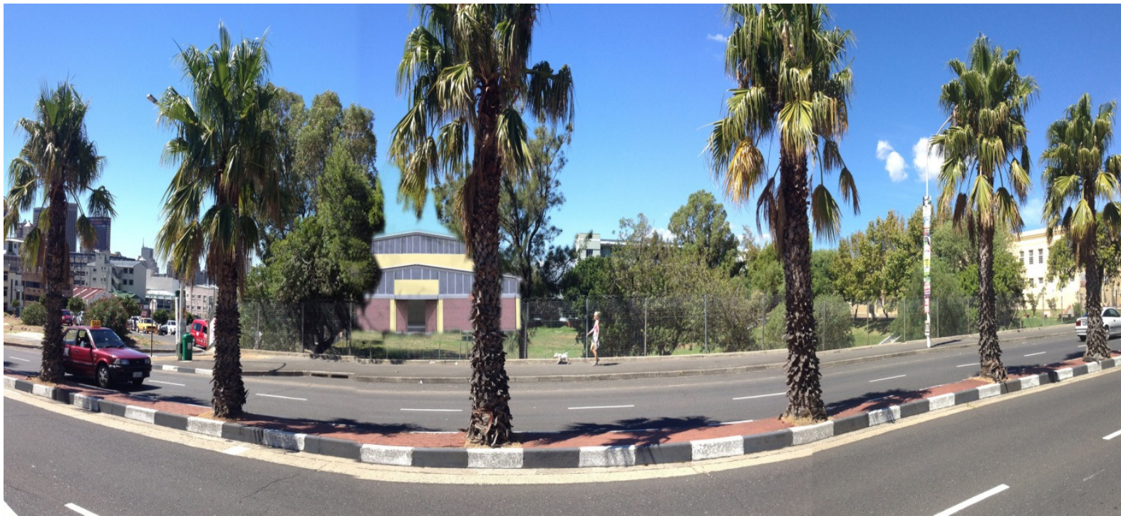
Figure 37: Artist impression multi-purpose hall along Roeland Street and Solan Road incorporating facebrick (ARM, Mowzer 2013)
