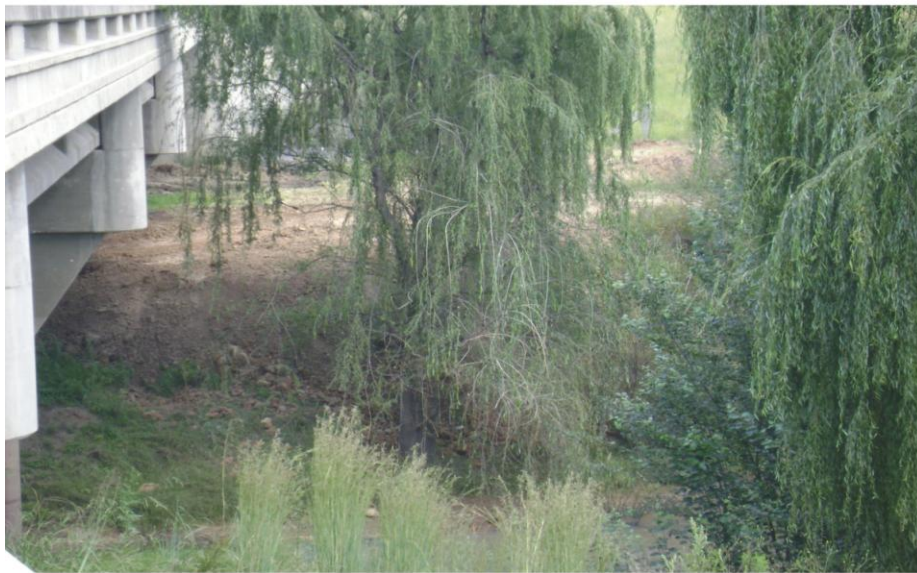
Figure 8. The N5 / Nuwejaarspruit Bridge, looking west. Construction of an additional passing lane will affect sedimentary bedrock, intact alluvial sediments (Quaternary) and recent topsoils.
