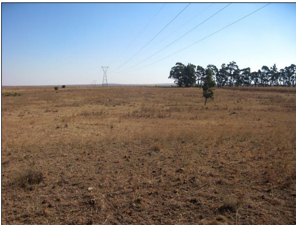
Figure 9. View to the northwest along the existing Harrismith-Sorata 132 kV line near Westlands farmstead. The raised terrain here mantled in reddish-brown rock rubble is underlain by a dolerite intrusion.
