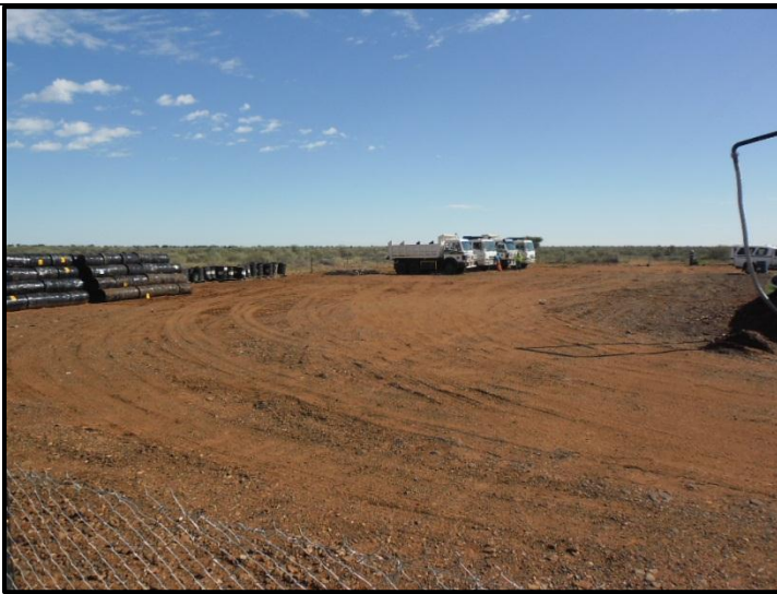
Figure 6. Existing construction camp.
