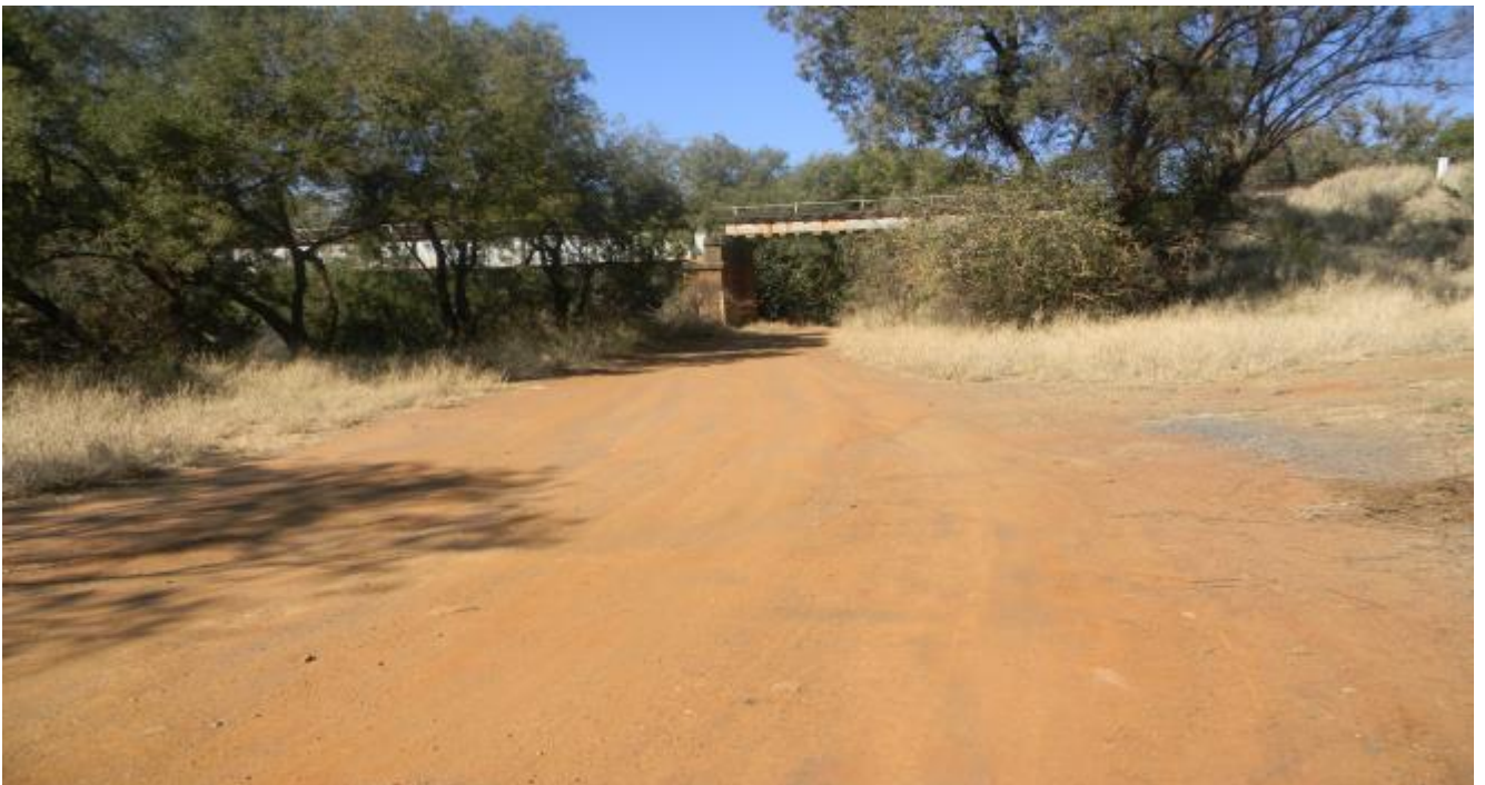
Plate 18: Photo 18: View of an access road that marks the eastern boundary of the proposed development site (Photograph © by Author 2016)
