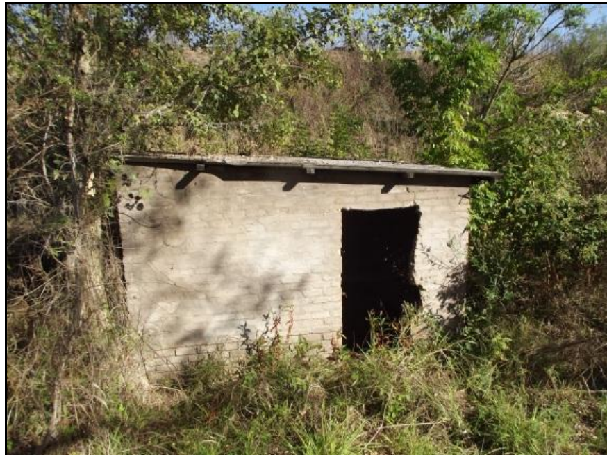
Fig. 8. Site H 4. Another pump station further east from site H 3.
