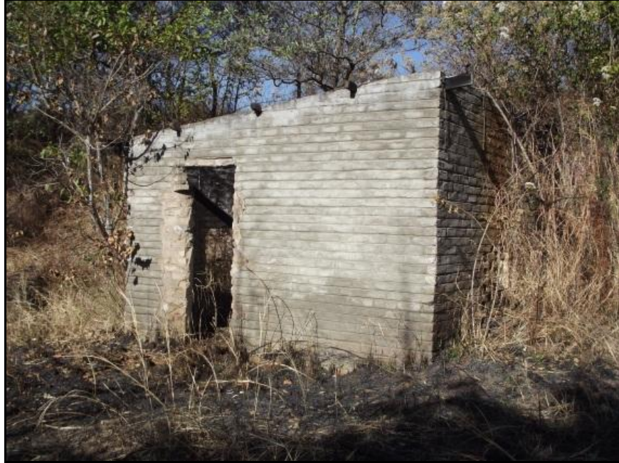
Fig. 7. Site H 3. An old pump station.
