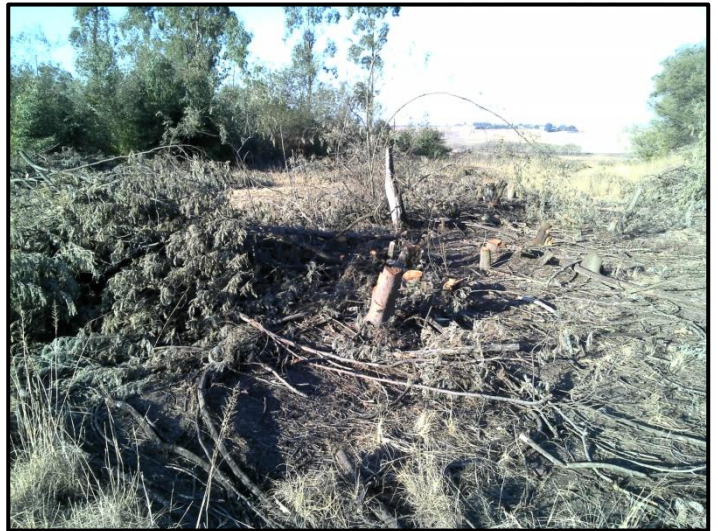
Figure 6. Clearing of trees.
