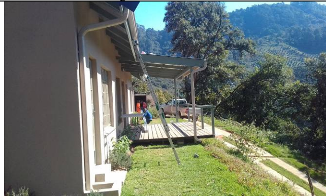
Fig 3: View of cottage
