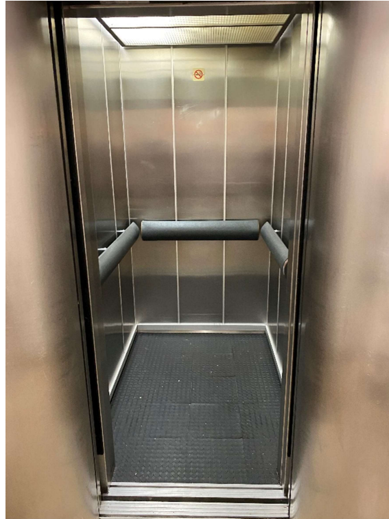
Figure 4: Lift to the Upper Kitchen from the Loading Area
