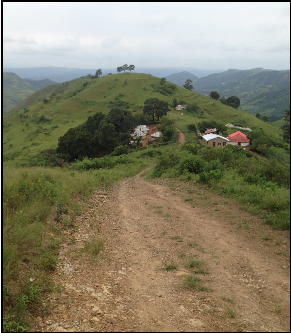
Figure 6. Photograph of the existing track to be upgraded as the Mqangqala Access Road.
