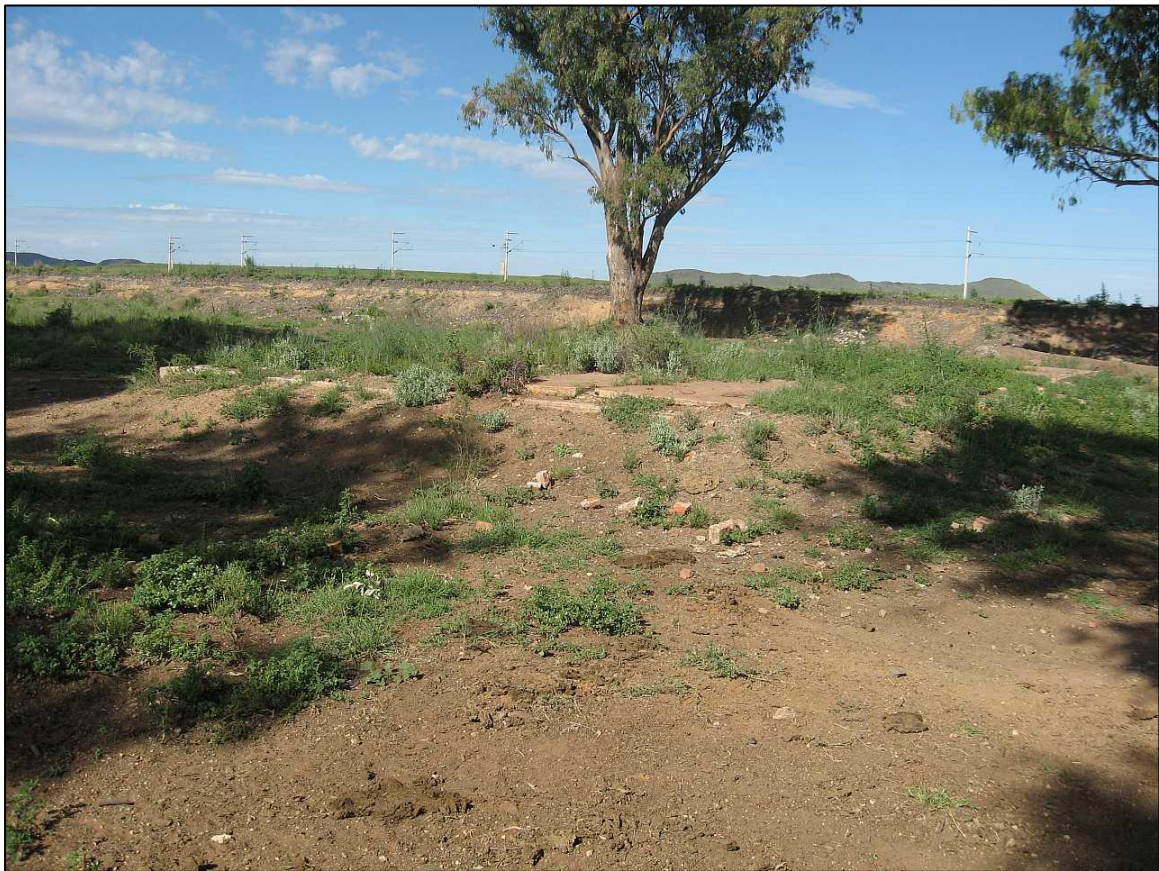
Figure 21: View of old railway structure
