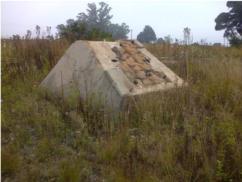
Figure 8: Headgear "feet"/pedestals.
