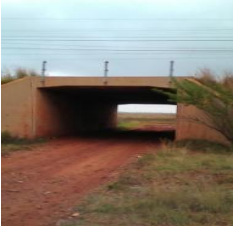
Figure 13: Old bridge on haul road.
