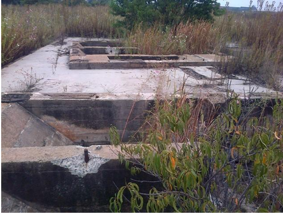
Figure 7: Old Headgear foundations.
