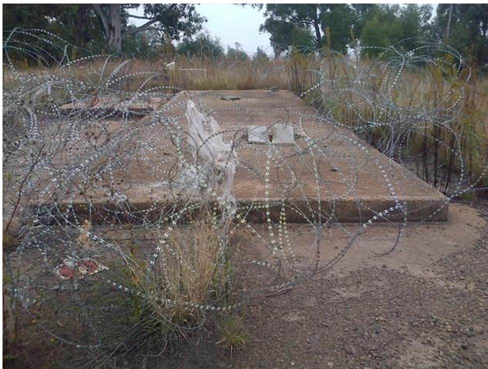
Figure 6: Old Holfontein Shaft.
