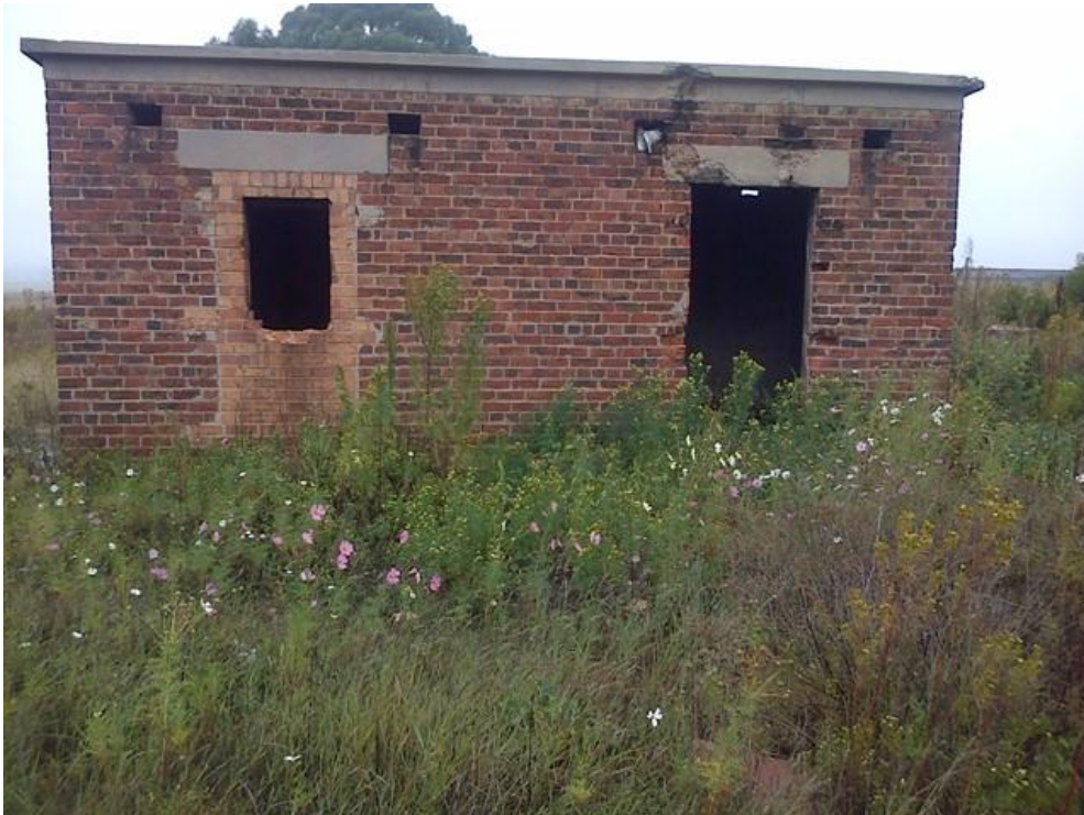
Figure 10: Old cement & brick building on Holfontein site.
