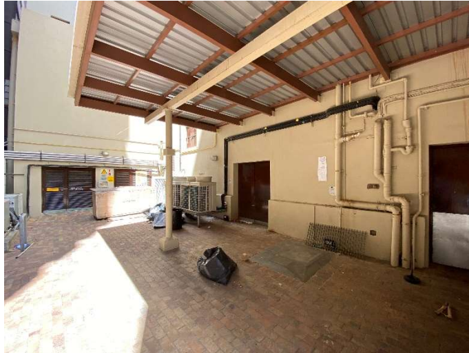
Figure 2: Service yard shared with the Marks Building
