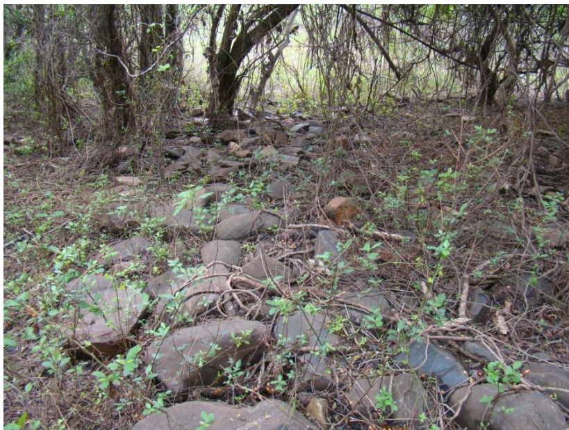
Fig. 58: The LIA stone wall is damaged by alien vegetation.
