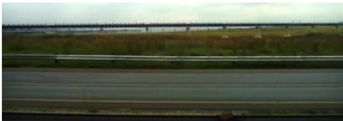
Fig. 17. The large sewer line bridge as seen from marker 2. (Google Earth image 2018.)
