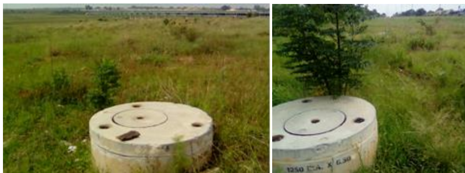
Figs. 15 and 16. Left. The view from marker 3 to marker 1. Right. The second of the two manholes at marker 3. (Photo's S.M. Miller, February 2019.)
