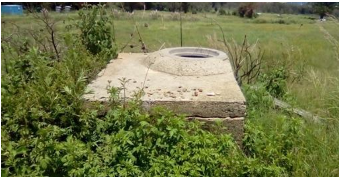
Fig. 84. Manhole between markers 1 and 2. (Photo S.M. Miller, February 2019.)
