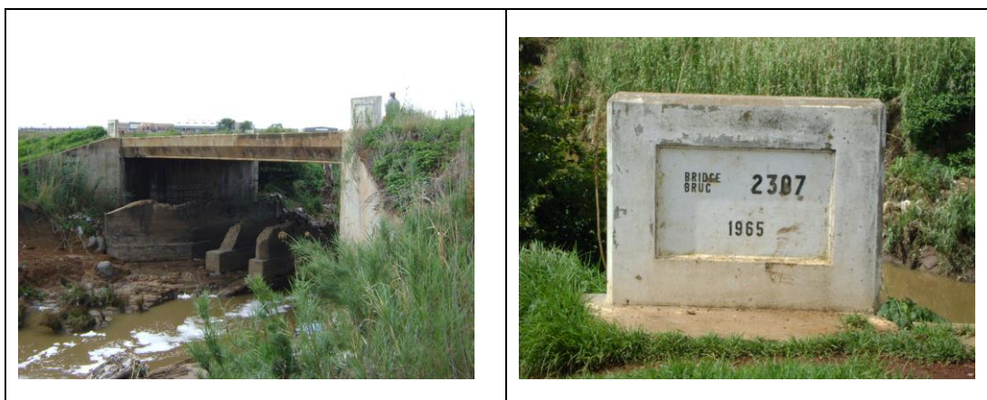
Fig. 8. The old road bridge.
