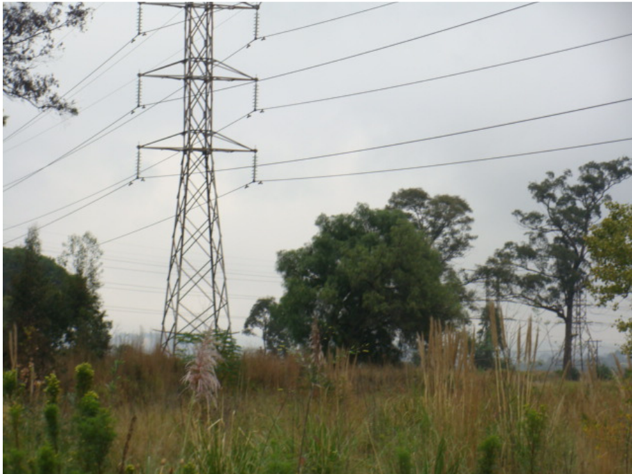
Figure 6: General view of the surveyed area including power lines.
