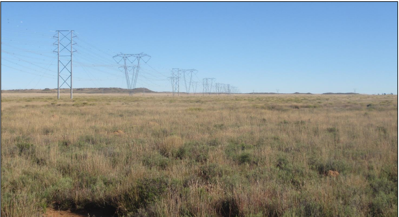
Figure 8: View towards the southwest along the southern part of the PV1 Alt. 1 corridor.
