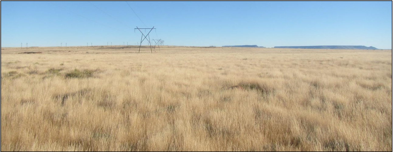
Figure 9: Looking towards the north along the northern part of the PV1 Alt. 2 powerline route.
