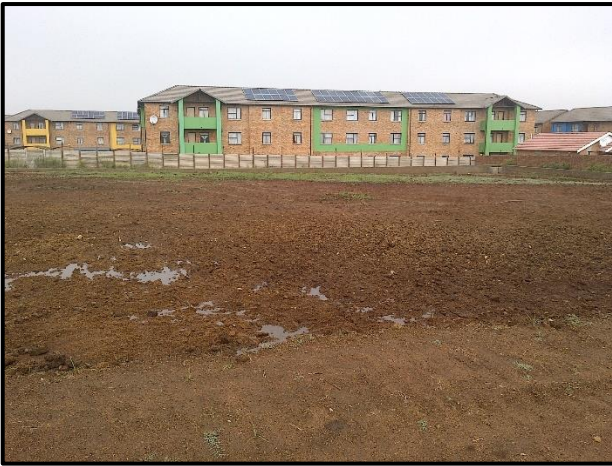
Figure 7.5. Existing excavations in the study area.
