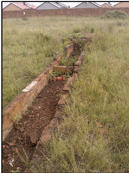
Figure 7.4. Demolished water trough.
