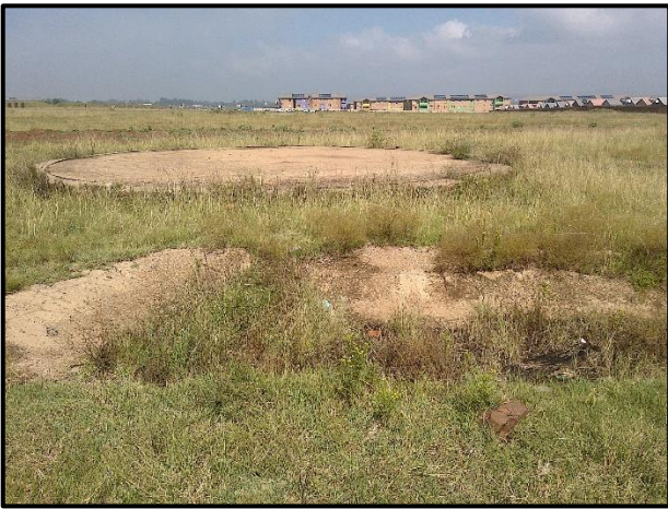
Figure 7.3. Demolished water reservoir.
