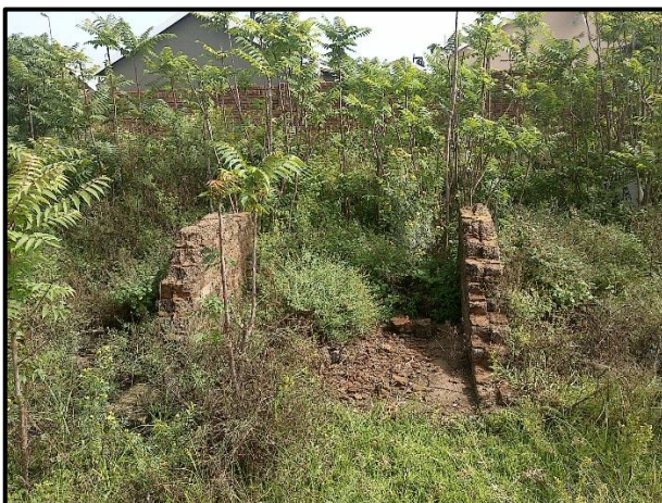
Figure 8.4. Demolished ruin at waypoint 306.
