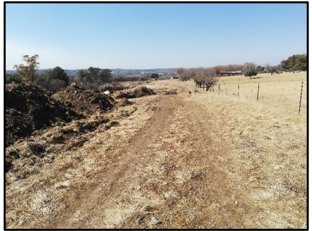
Figure 17. General site conditions – Access Road B.
