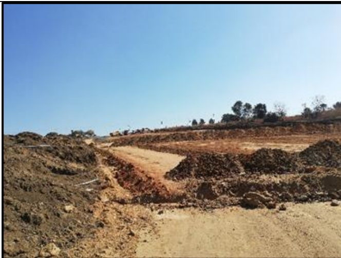
Figure 7. General site conditions.
