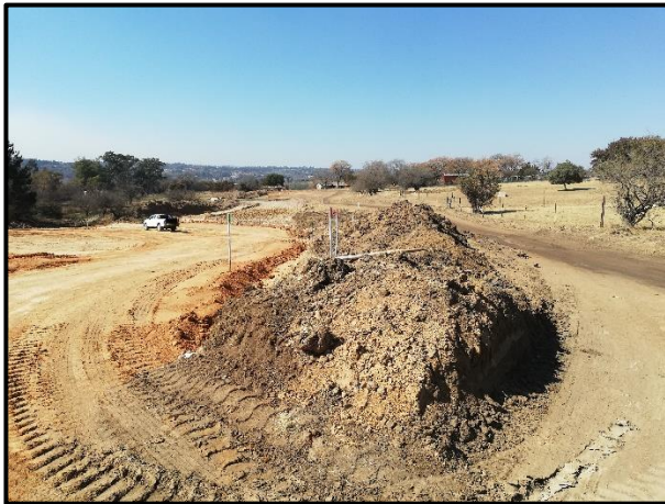
Figure 16. General site conditions – Access Road B
