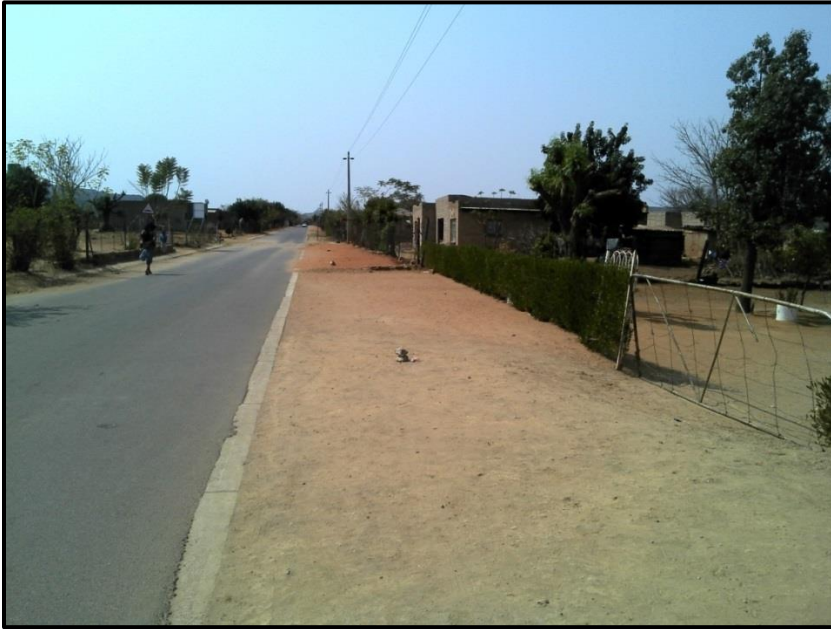
Figure 8. Existing road at the Bakenberg section.
