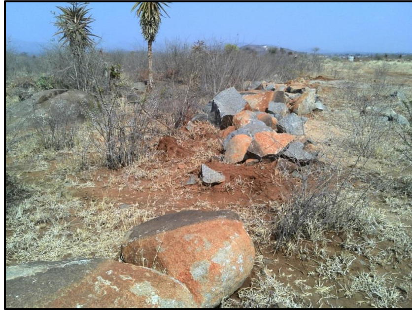
Figure 9. Existing pipeline construction activities in the Tshamahansi section.
