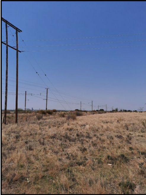
Figure 7.1. Existing Powerline infrastructure.
