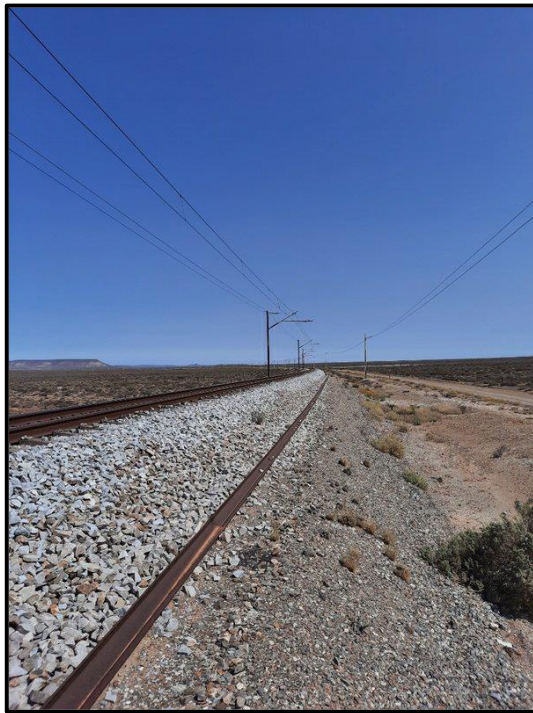
Figure 7.4. Existing railway in the study area.
