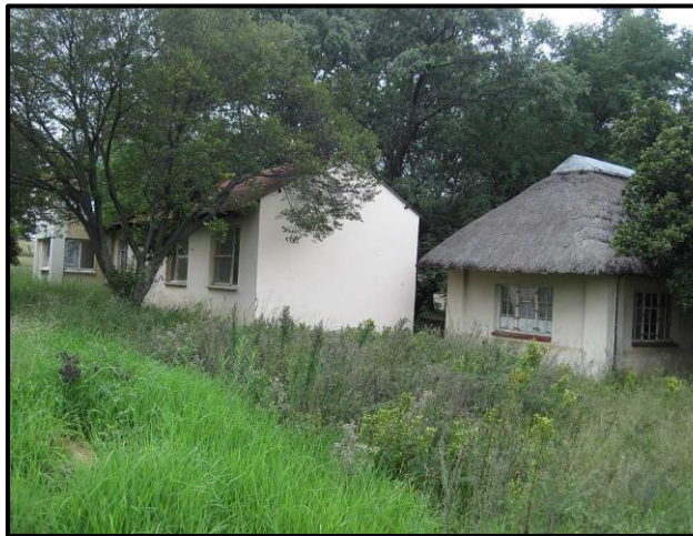
Figure 16. General site conditions- Existing structures
