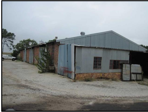
Figure 14. General site conditions – existing structures
