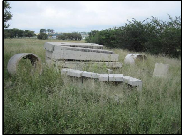
Figure 13. General site conditions - dumped material
