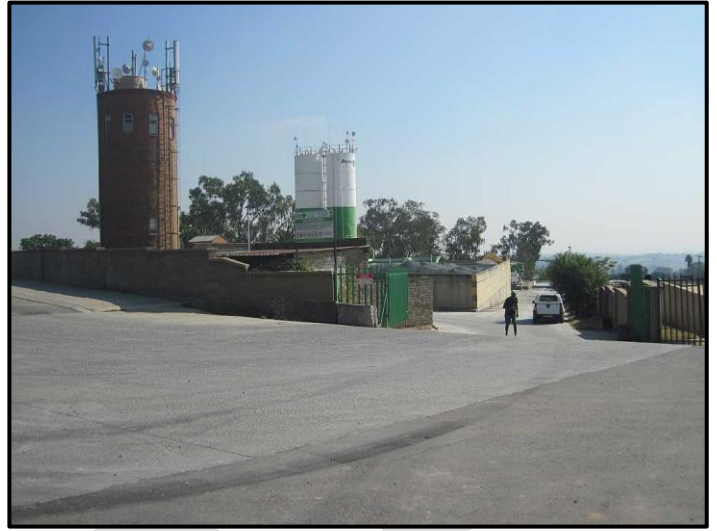
Figure 12. Cement facility bordering the site.
