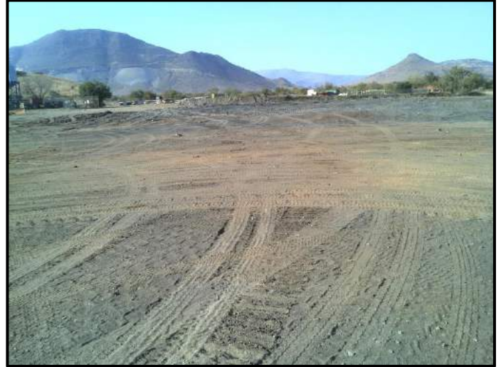
Figure 7. Cleared areas at North Shaft.
