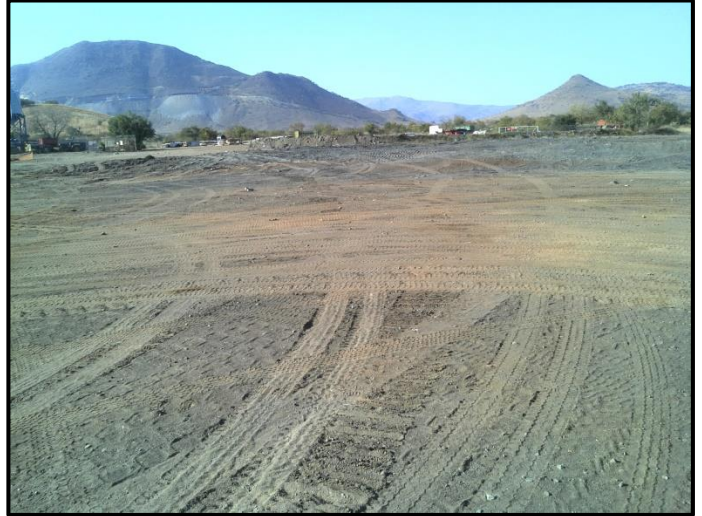
Figure 7. Cleared areas at North Shaft.
