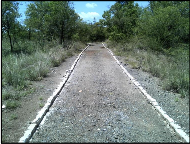
Figure 6. Existing roads at the Met grade expansion area.
