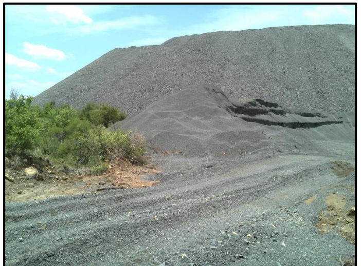
Figure 13. Discard dump expansion area general site conditions.
