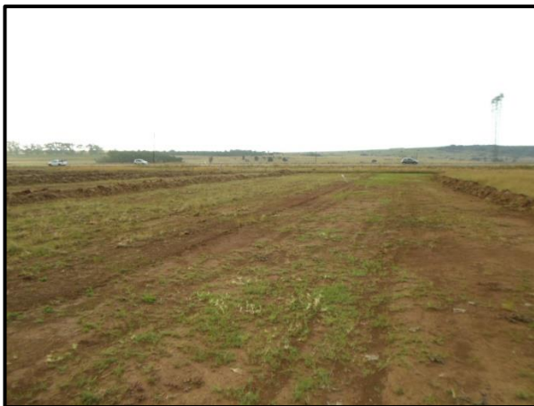
Figure 16. General site conditions.
