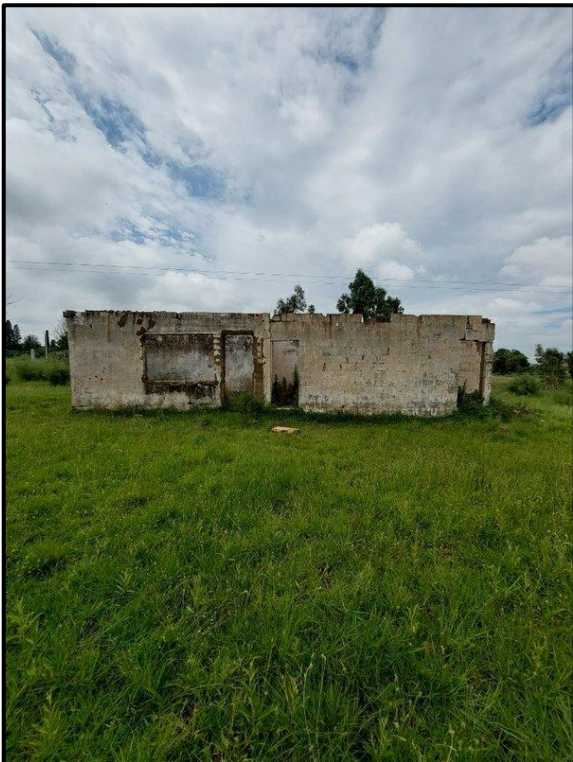
Figure 8-12. North facing wall of the structure at EF003.
