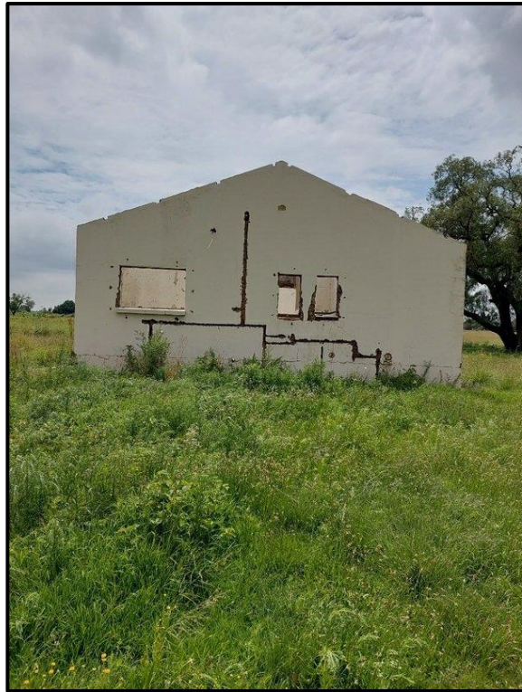
Figure 8-35. West facing wall of the secondary house at EF009.
