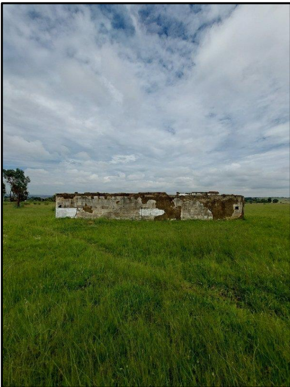
Figure 8-4. East facing wall of the structure at EF001.
