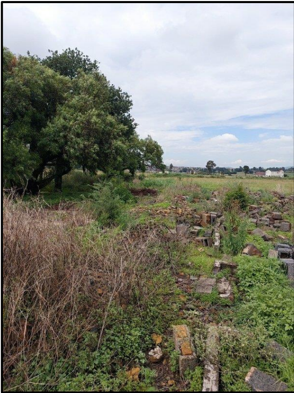
Figure 8-18. View of the foundations and various cement bricks that seem to have been recovered. Image facing west at EF004
