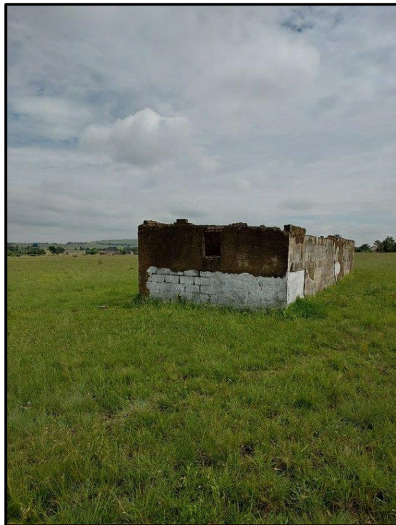
Figure 8-5. South facing wall of the structure at EF001.
