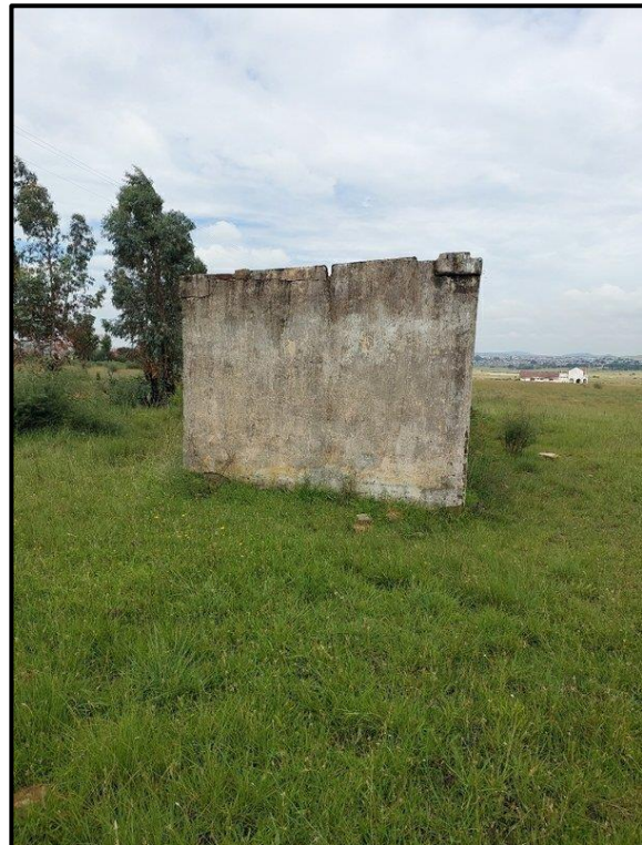
Figure 8-13. East facing wall of the structure at EF003.
