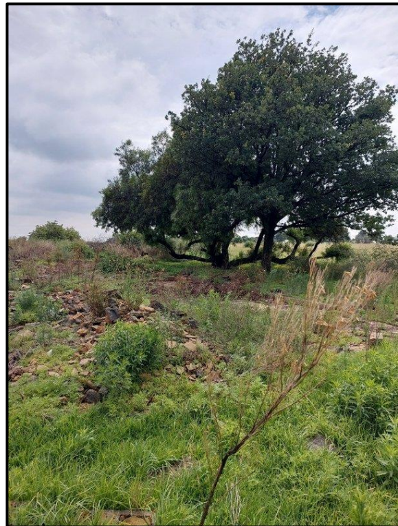
Figure 8-17. Alternate view of the demolished structures showing a row of trees running along the edge of the site at EF004.
