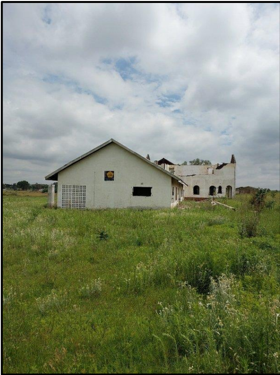
Figure 8-30. South facing wall of the main structure at EF009.
