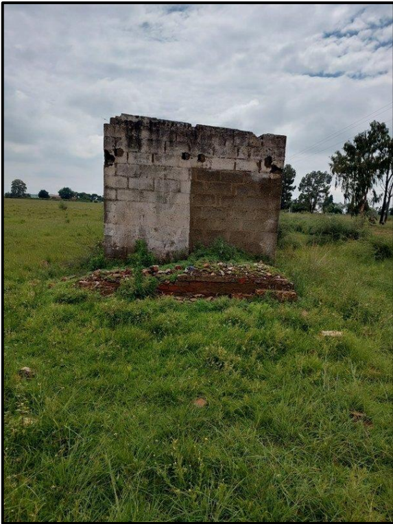
Figure 8-14. West facing wall of the structure at EF003.
