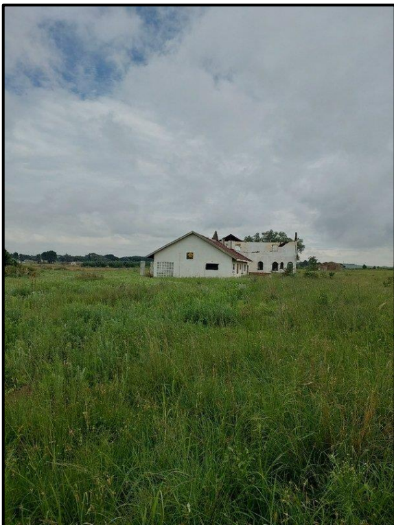
Figure 7-3. Various degraded structures are scattered across the proposed project area.
