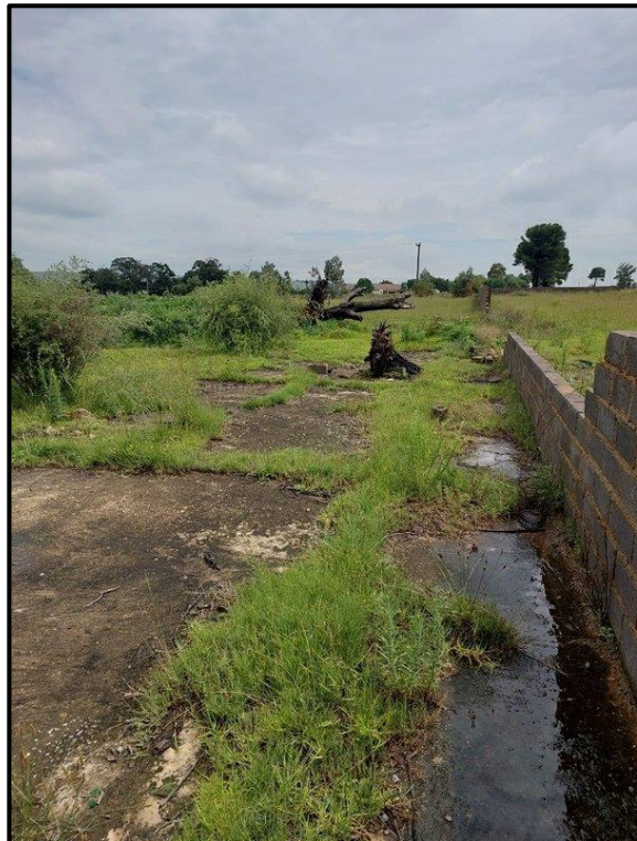
Figure 8-9. The foundations are situated along an existing wall at EF002.
