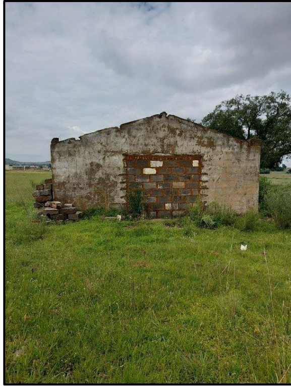
Figure 8-39. South facing wall of the garage structure at EF009.
