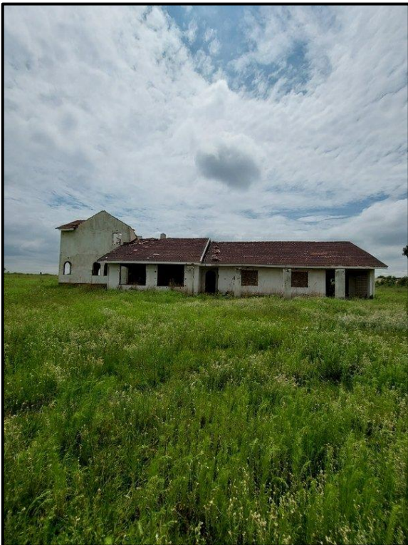
Figure 8-32. West facing wall of the main structure at EF009.
