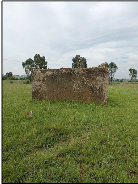
Figure 8-3. North facing wall of the structure at EF001.
