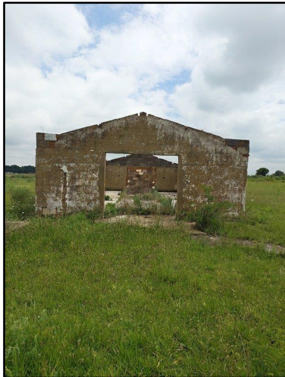
Figure 8-37. North facing wall of the garage structure at EF009.
