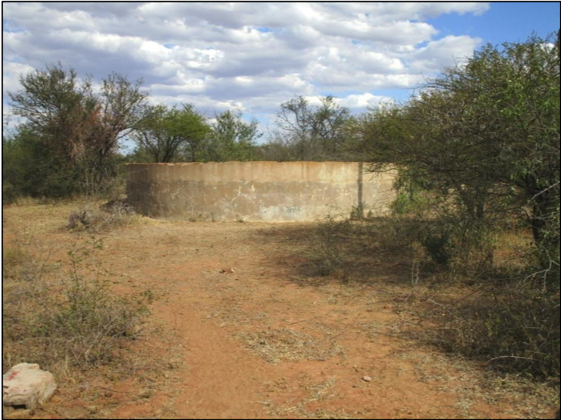
Figure 12. View of reservoir at feature 15.
