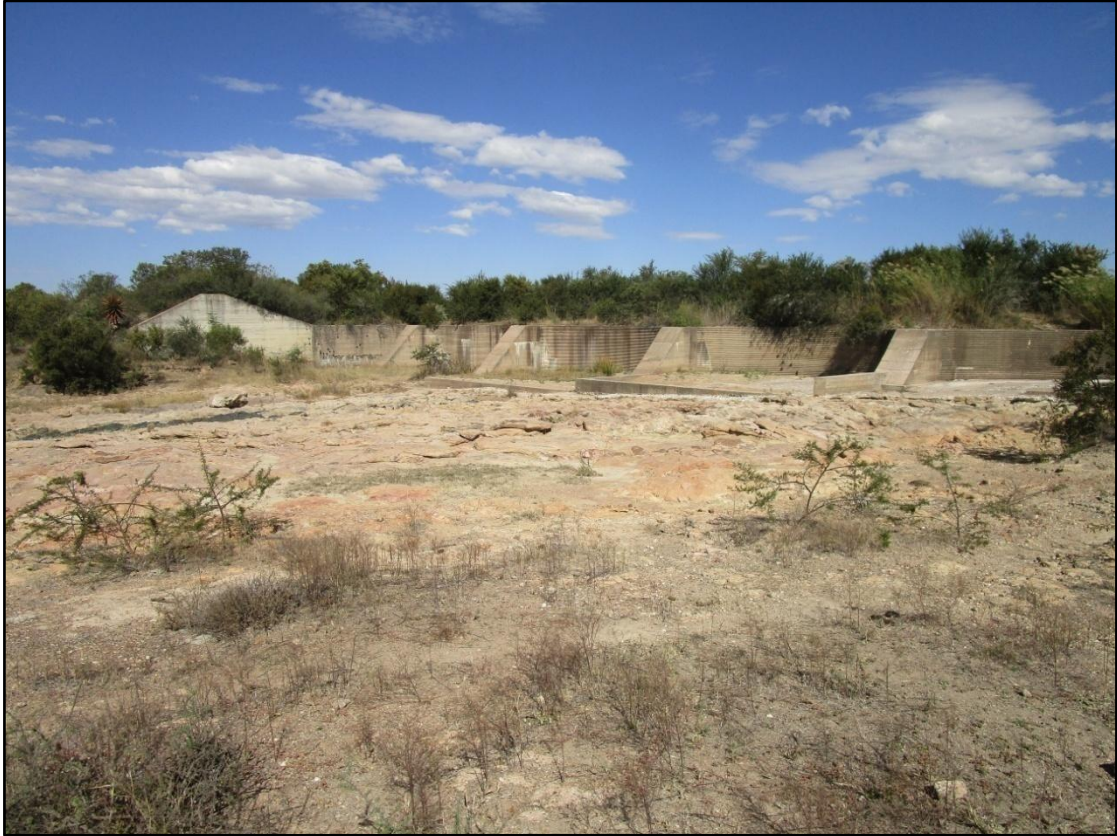
Figure 10. View of weir at feature 13.
