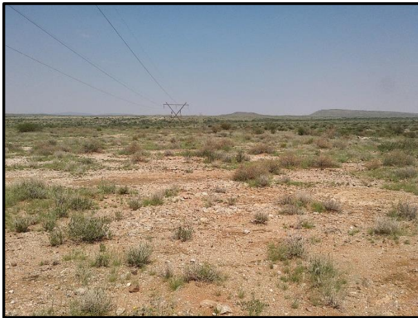
Figure 8-1. Existing powerline infrastructure in the study area.
