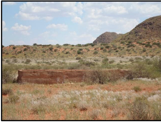
Figure 8-4. General site conditions at waypoint 456.
