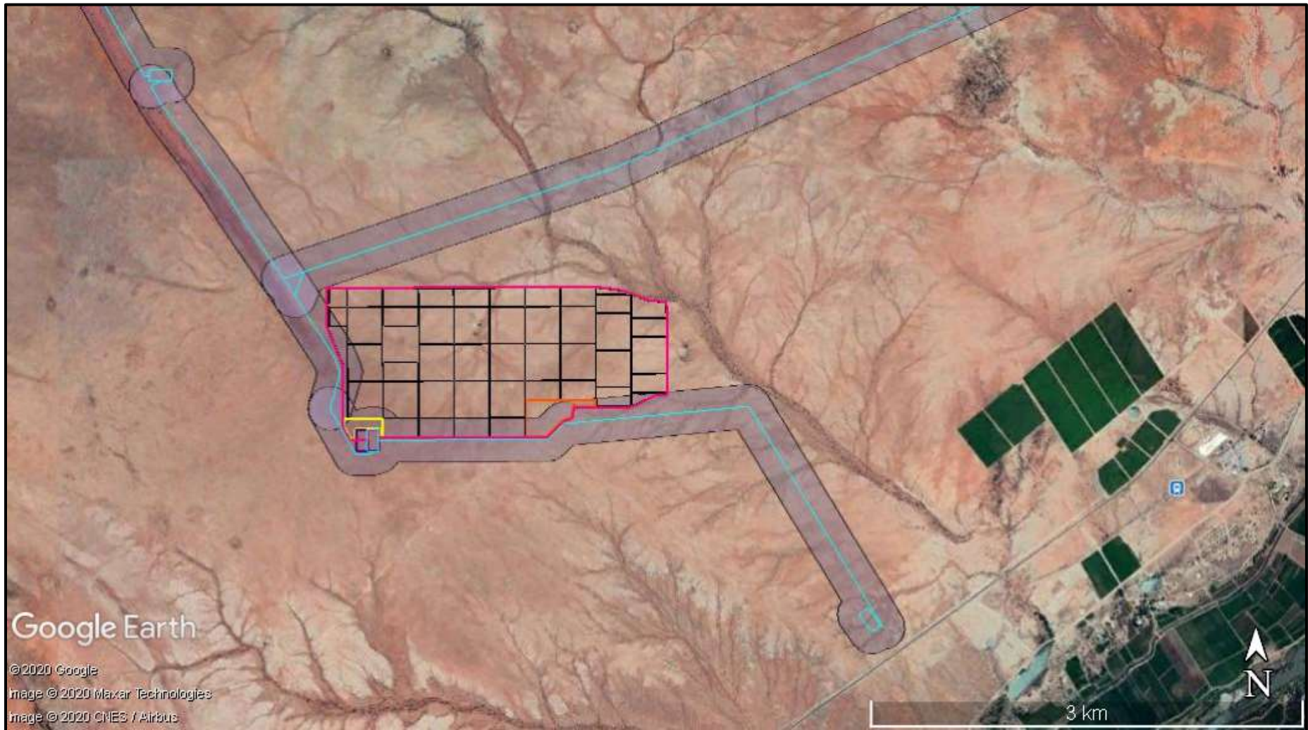
Figure 3. Satellite image indicating the proposed PV layout and powerline grid corridors (the grid is only for contextual purposes and is addressed in a separate BAR) (Google Earth 2019).
